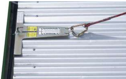
Sit the anchor on top of corrugation roofing iron as shown
