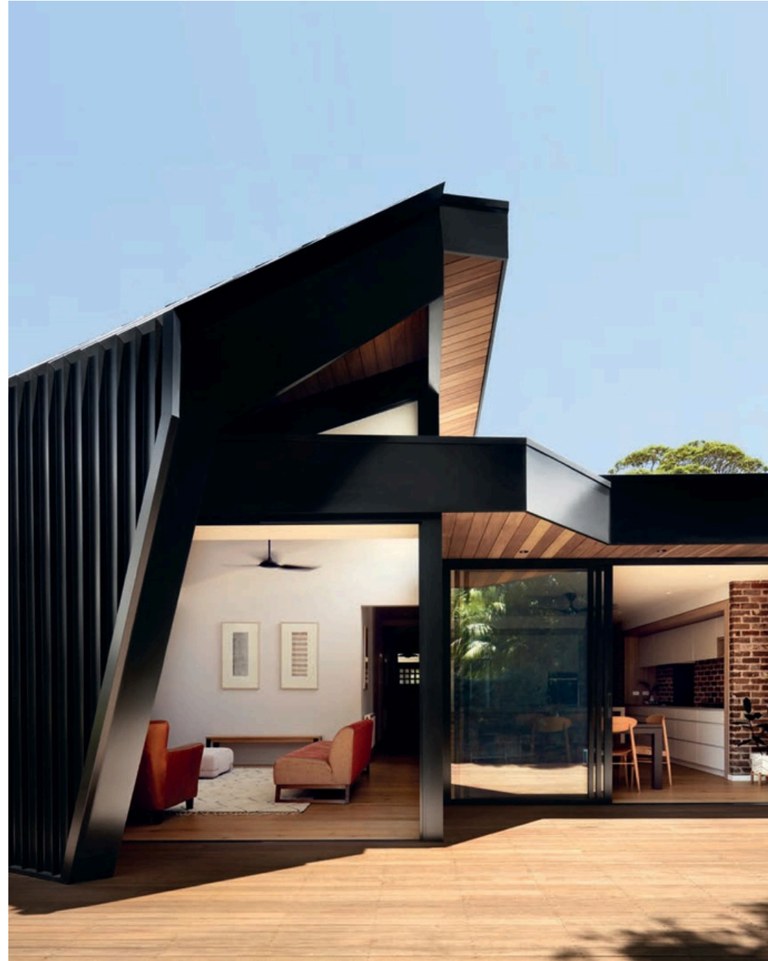
• Roofing and walling | COLORBOND® steel Night Sky® in a Classic finish.
