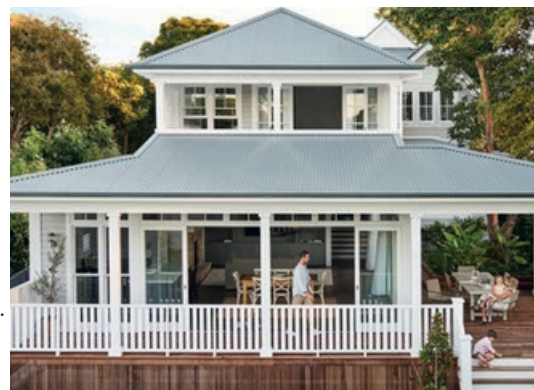
• Roofing and gutters | COLORBOND® steel Ironstone® in a Classic finish.
